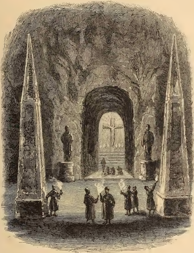
AN UNDERGROUND CHAPEL.
